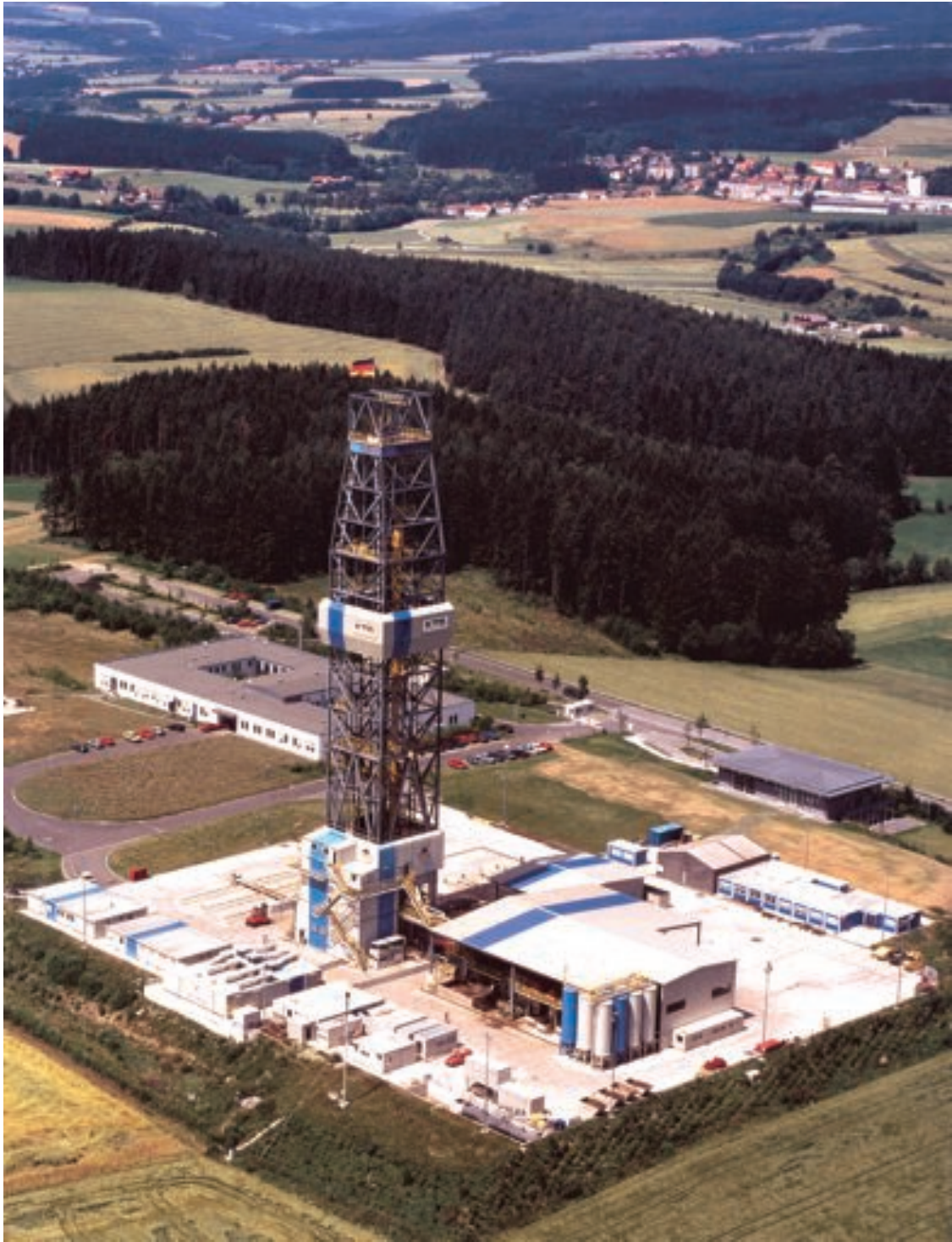
KTB (Kontinentale Tiefbohrung, Continental Deep Drilling, Depth: 9101 m) The drilling rig at Windisch-Eschenbach (Bavaria, Germany) (Foto: KTB-Archive).
