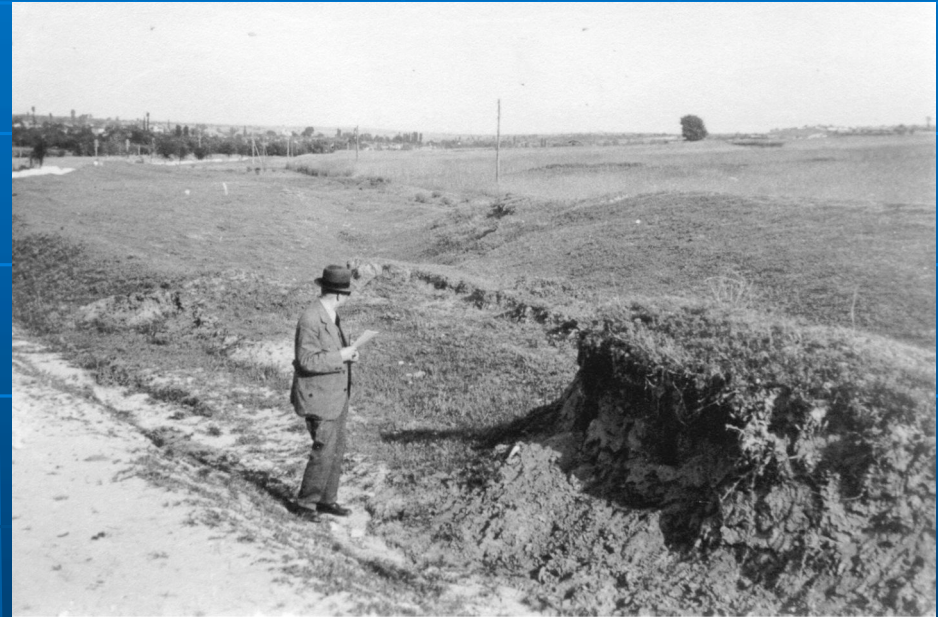
29.04.1939. Fracture near Papazli - 11 year after the earthquake
